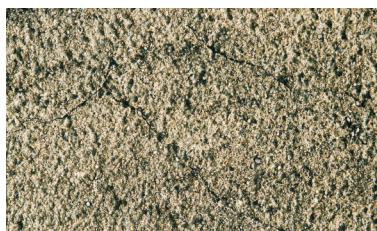
Existing render with cracks
