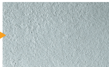
Base coat/bridging of the existing coating with KEIM Contact-Plus
